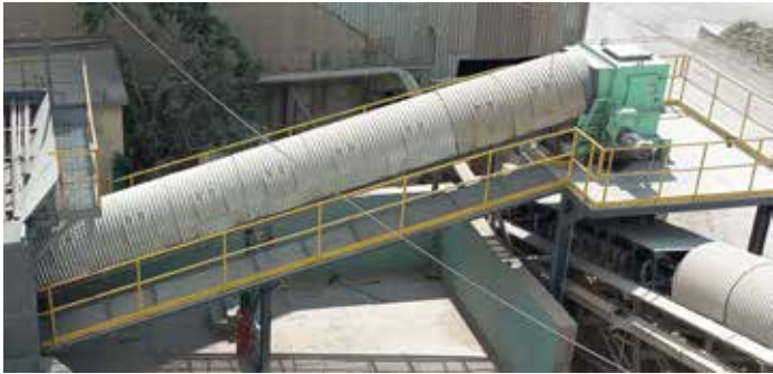
JAM: New Iron Ore Hopper
