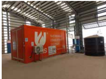
JAM: Transformer and UTI's
