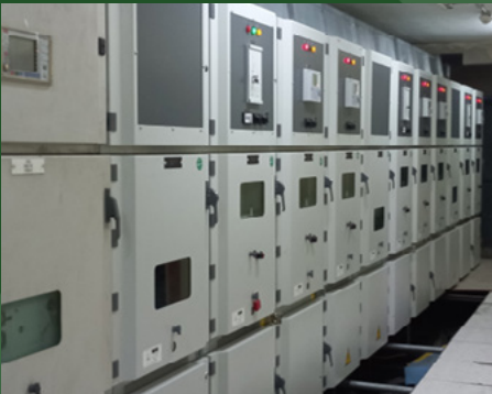
Replacement of Switch Gear TR4
