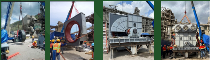
Assembling a 4500 HP Motor for Cement Mill 4
