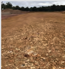
Toco highway sub-base – proving limestone aggregate can be used as a sub-base development in road paving
